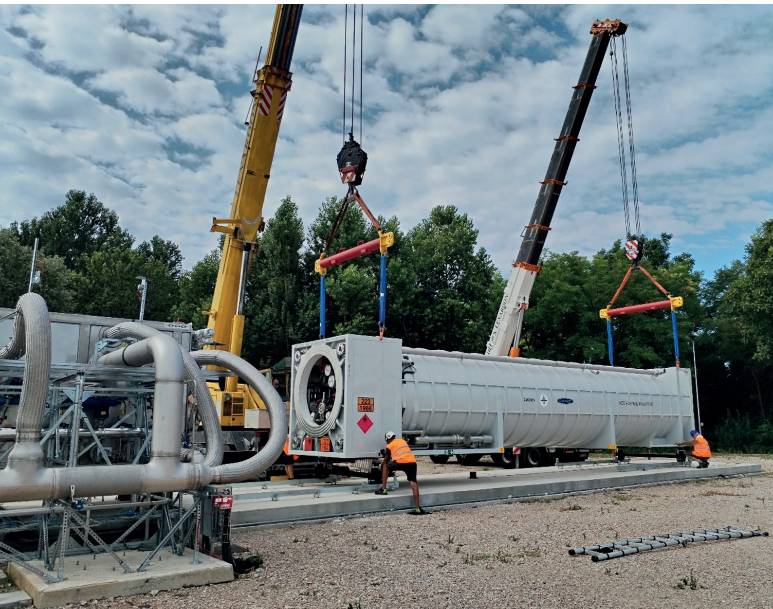
Figure 4: Installation work: the LH2 storage tank is lifted into position
