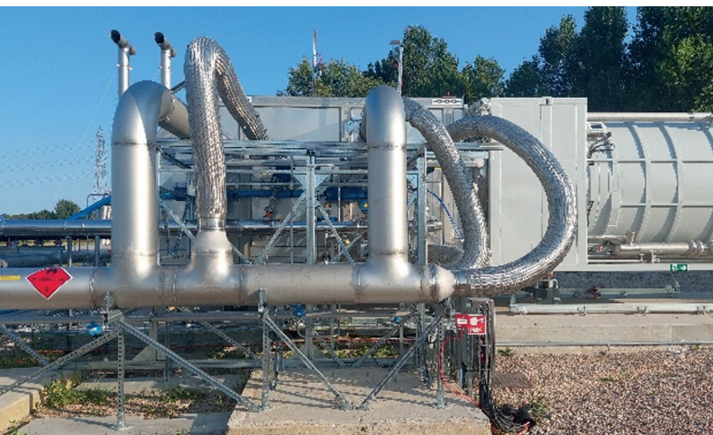
Figure 1: Monitoring the system during testing
